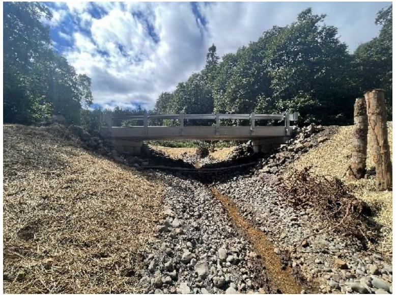
After: Clear-span bridge restoring fish passage Photo credit: ODF
